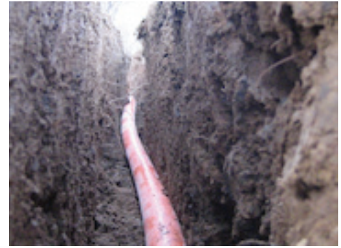
Trench installation of a FiberPatrol X in-ground sensor.
